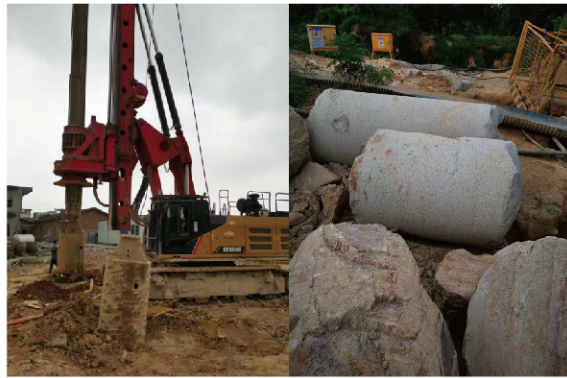
• Construction site in Fujian Putian
