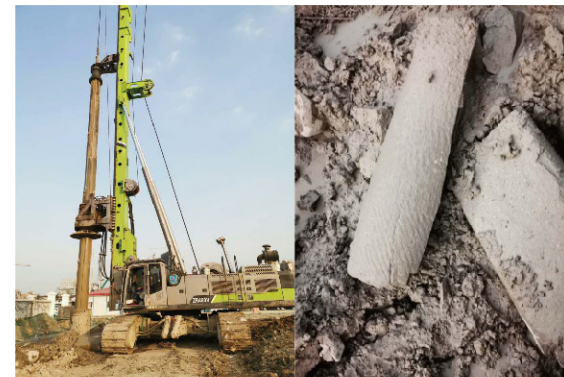
• Construction site in Suzhou Mudu
