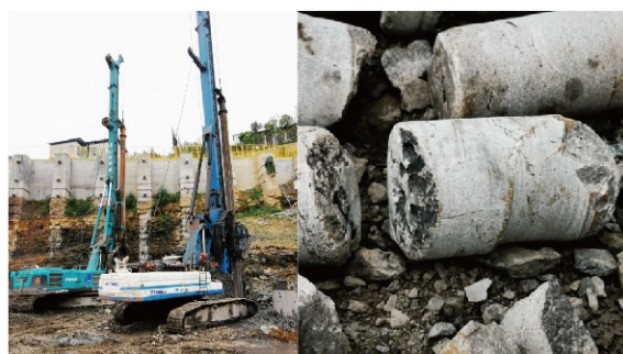
• Construction site in Chongqing
